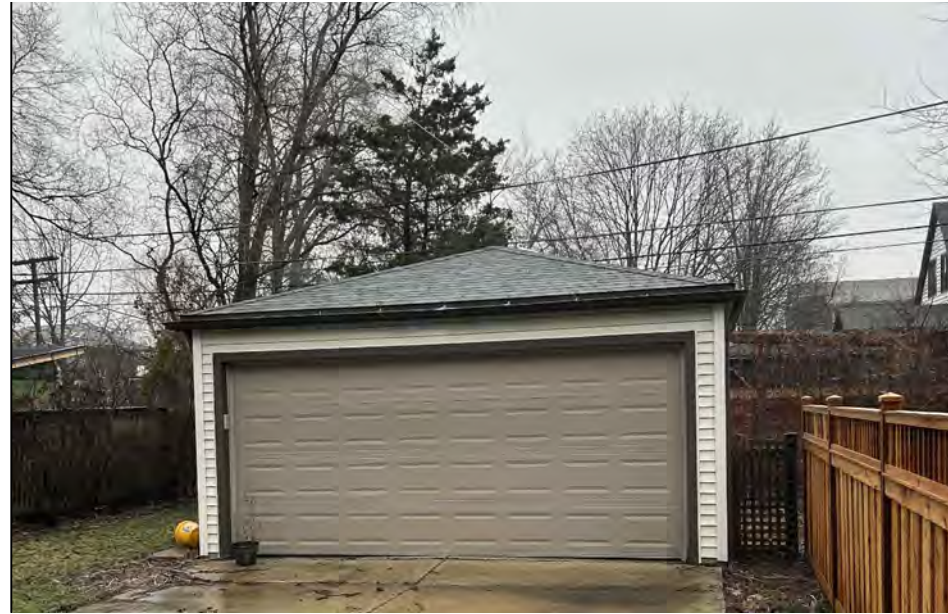
PROPERTY TO THE NORTH (613 N HARVEY AVE.)
