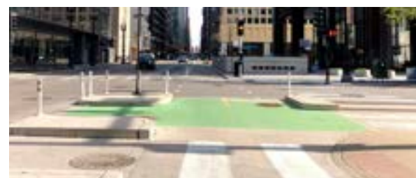
Example of a protected intersection.
