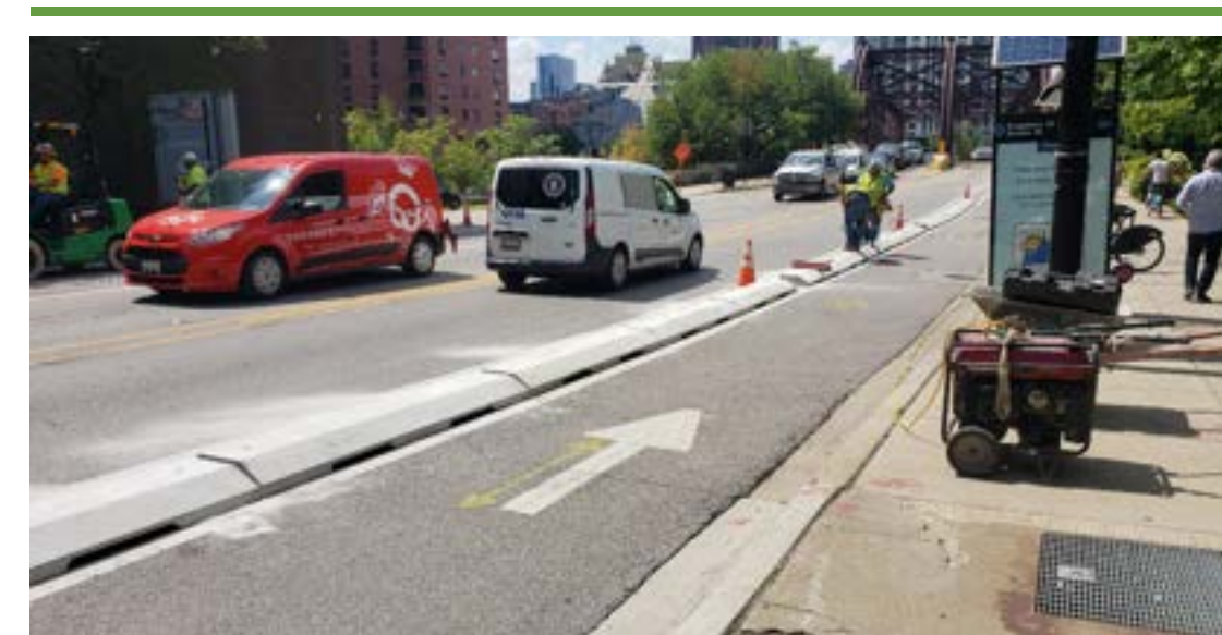
Installation of pre-cast curbs to form a protected bike lane.
