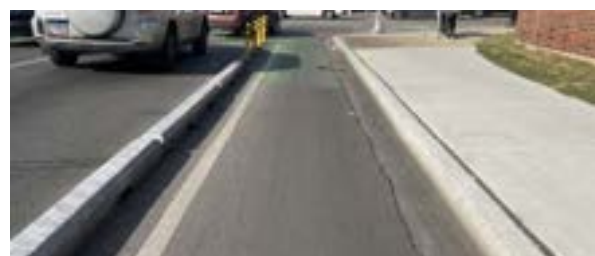
Example of pre-cast concrete curbs
