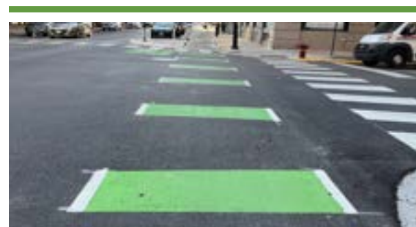
Green conflict markings through an intersection.
