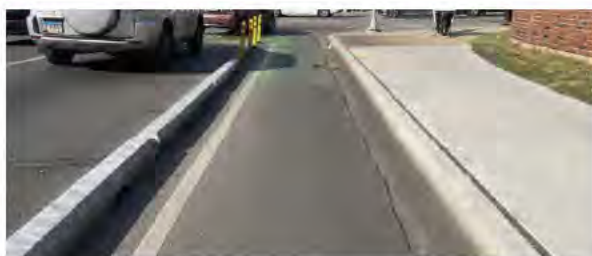
Example of pre-cast concrete curbs
