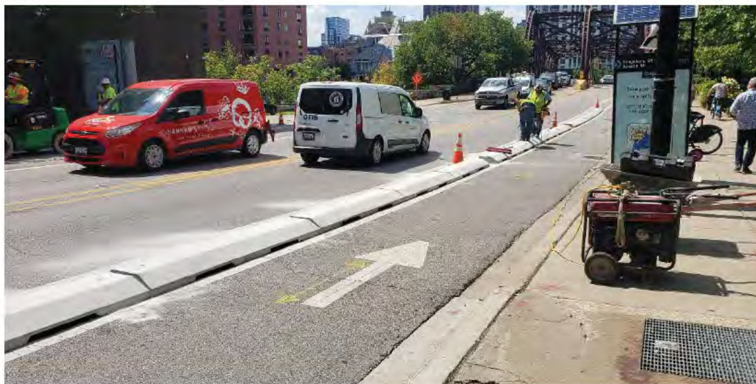
Installation of pre-cast curbs to form a protected bike lane.
