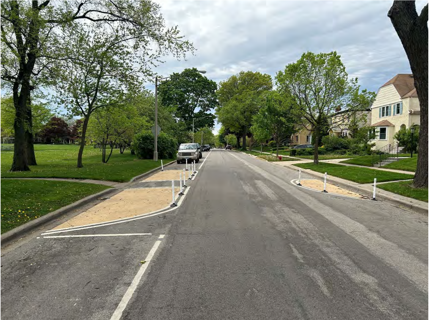
Figure 3. Paint and Post Pinch Point Example
