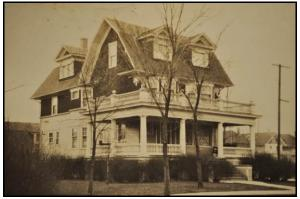
Historic photos were also vital in the design and reconstruction of the original open front porch. All of the wood siding and wood shingles were repaired or replaced as need, stripped and repainted.
