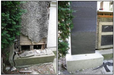
Finally, stucco on the main house façade required repair, removal and replacement where necessary. New backing was inserted where needed, and all the paint was stripped from the surface. All wood trim and wood windows were stripped and repainted, and all stucco was painted and coated. The result is an incredible transformation not only for the house, but also for the surrounding properties and the block.
