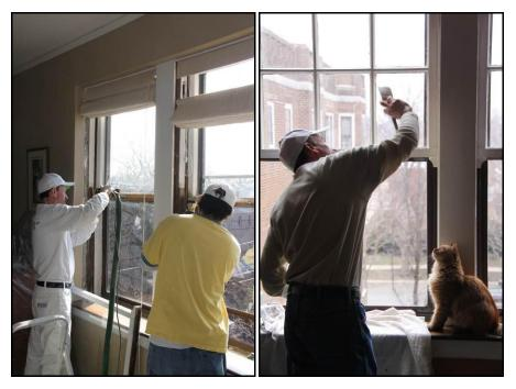
All existing metal storm windows were removed in order to scrape and strip the windows and sills, conduct repair work, then prime and repaint the windows. The storm windows were reinstalled after the work was complete. Individual unit owners determined whether the additional repair and interior painting would be done.
