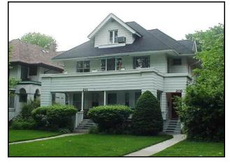
The project involved removing all of the aluminum siding off the front façade and front porch of the house and restoring the stucco siding and wood trim based on the original drawings in possession of the owners. This allowed Fortune Restoration to recreate the center dormer window and match the stained glass design of the smaller windows which had been covered.
