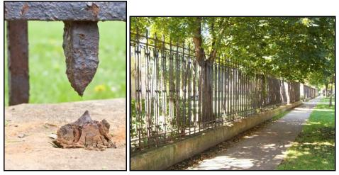
The work included careful removal of the fence panels on the north and east sides of the park, and restoration and painting of the panels offsite, including the removal of existing paint, rust and scaling. Midwest Fence then repaired the fence and replaced some deteriorated pickets and other components to match the original. Following stripping and repair, the fence was primed with a zinc-rich primer and painted with a high performance epoxy coating.
