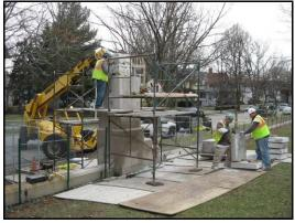
Upon completion, the restored steel fence panels were set on the limestone plinth. Existing holes in the plinth were reused and filled with non-shrink grout to securely fasten the fence.
