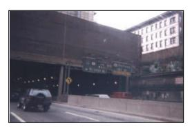
• Cut and cover expressway, with apartments and bus terminal built on top
