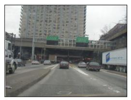
Originally constructed as a two-lane bypass, the expressway now carries more than 250,000 vehicles per day on its 12 lanes of roadway. The original 178th Street and 179th Street tunnels were designed in traditional Moses-style, utilizing stone-faced arch portals and "Whitestone" lightposts. Viaducts with single circular supports that connected the tunnels with the Washington (Heights) Bridge are still in use today.
