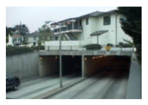
**Fig. 3a:** Lighthouse Ave. Tunnel – has extensive pumping / collection storm water system due to below sea
