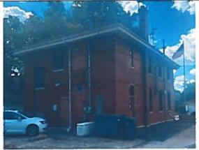
Fire Station #2 – Looking SE – Note Small Windows Located in Large Sections of Newer Brick Infil & Infilled Areas Where Windows Were Likely Removed
