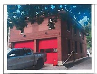
Fire Station #2 – Looking NW – Note Small Windows Located in Large Sections of Newer Brick Infil
